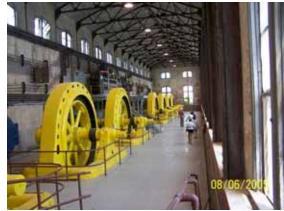
A view inside the plant, with its long hall and row of seven generators, which convert the waterpower produced by water flowing through turbines into electricity. Four of the generators are currently in operation; the rest will be brought on line shortly.
