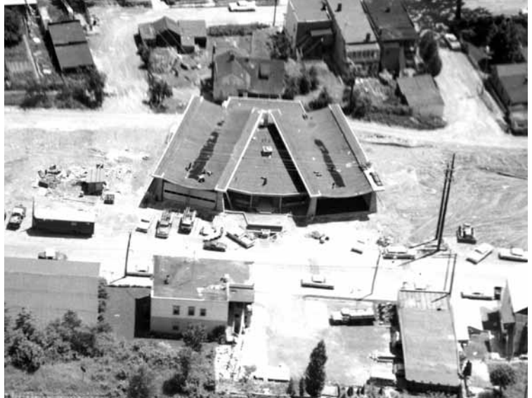
Construction of the Central Avenue Firehouse, June 1966. Bernard T. Shaw Collection.
