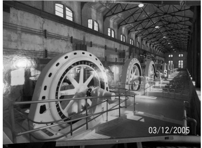
The restored Mechanicville hydropower plant, still generating electricity after more than 100 years.
